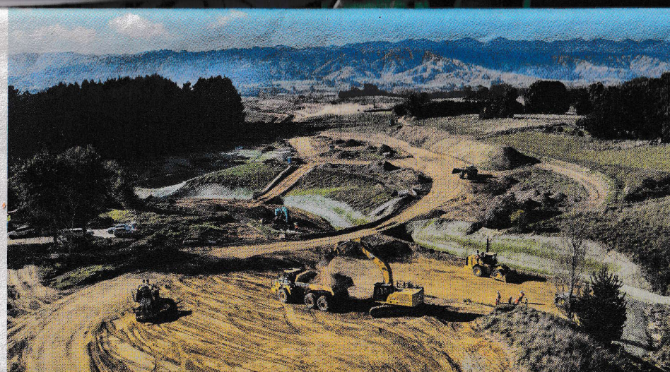
ABOVE: Earthworks underway near Sorensen's Rd as construction continues on the Ōtaki to north of Levin (Ō2NL) expressway project. The area has also been the focus of extensive ecological rescue work, including the relocation of native fish, eels and lizards. SUPPLIED
